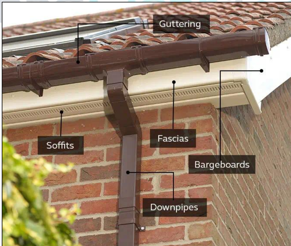
Image 2: Guttering components.
